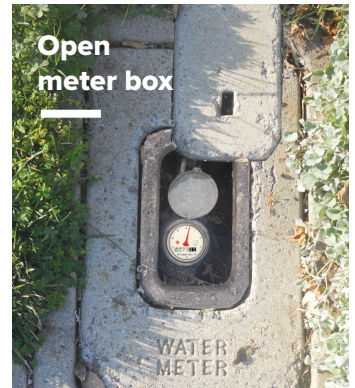
Meter number on meter cover
